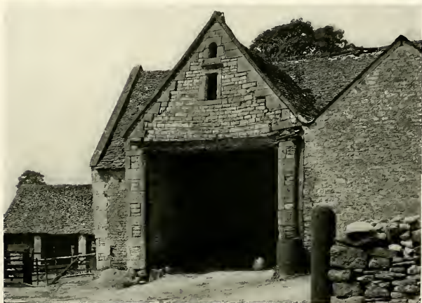
TWO VIEWS OF A BARN AT COTSWOLD HILLS The openings in the stone wall, admitting light and air into the building, are interesting
